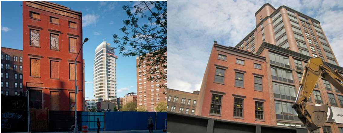
Before renovation and the construction of the 15-story rental apartment building next door After the construction of the building next door
